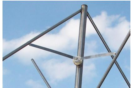
With an input rating of 3 kW per bay, the **TLV** is perfect for any low band VHF application. The low wind load and weight will allow mounting these antennas to smaller structures. And being half-wave spaced will leave a smaller RFR footprint on the ground. The excellent circular polarization that this antenna provides maximizes the reception possibilities for your viewers. So if you have a low band project coming up, the **TLV** antennas should be your first choice!
